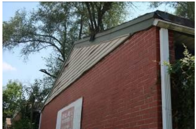
Siding Damage
