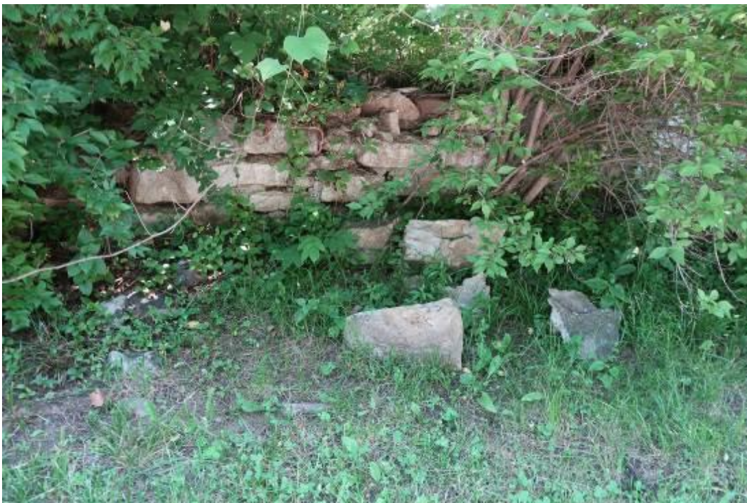
Collapsing Retaining Wall Along E 62 nd Street
