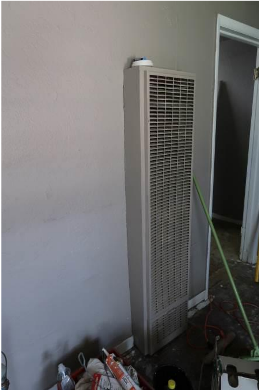
Wall Mounted Heating Unit (No Ductwork)
