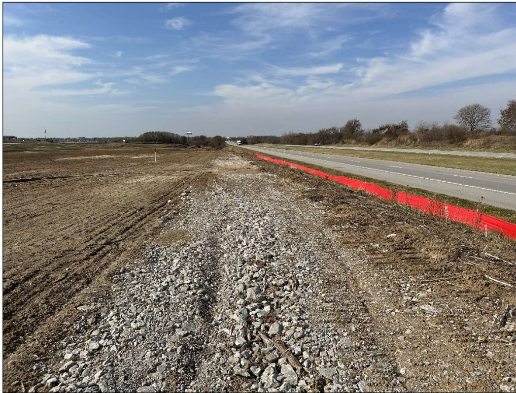
Looking northwest along north boundary of Study Area, Interstate 435 – crushed concrete as road base
