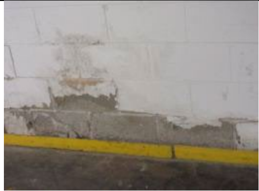
Dilapidated load bearing concrete retail parking Sheraton Garage.
